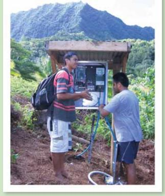
Avana streamflow station setting up instrument housing, bubble sensor and logging equipment. Note the steep mountains typical of Rarotonga.
